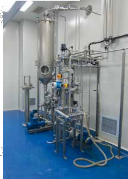
1-stage SIGMAVAP Evaporating Plant pharmaceutical products - evaporating capacity 500 kg/h
